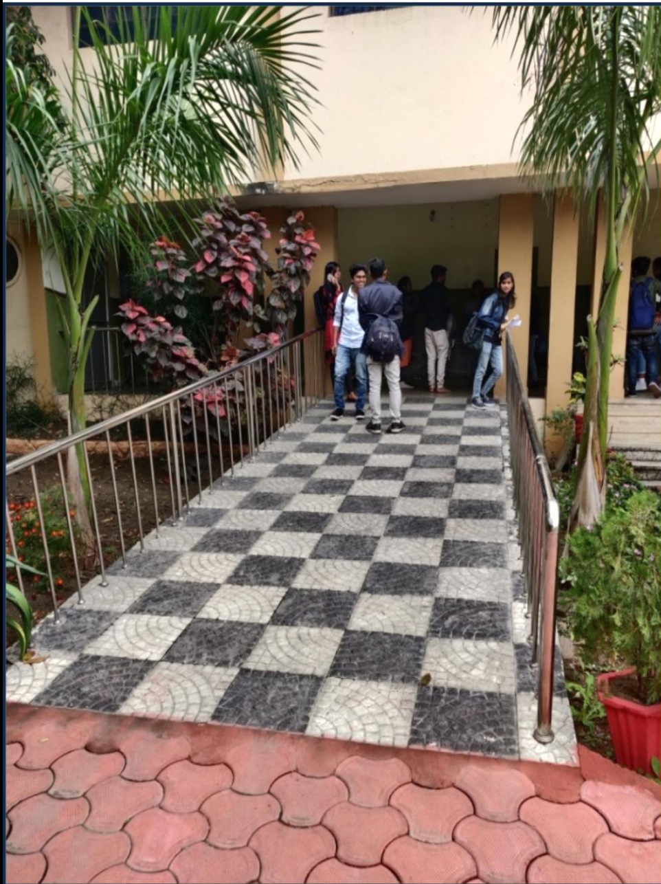
RAMP FOR EASY ACCESS TO CLASSROOMS
